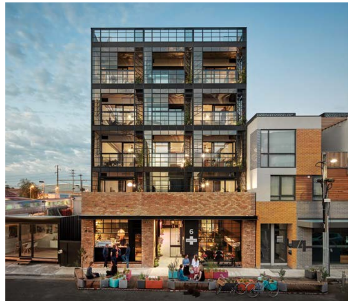
Nightingale 1 is an apartment building in Melbourne which activates the ground floor with a commercial studio space, seating nooks, a semi-public laneway, and a kerbside social space.
